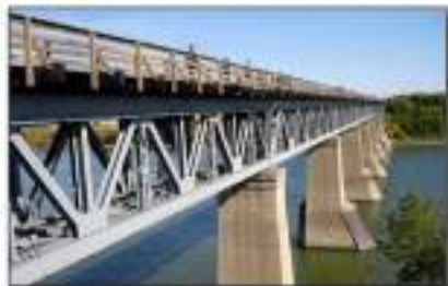
Saskatoon's Train Bridge
